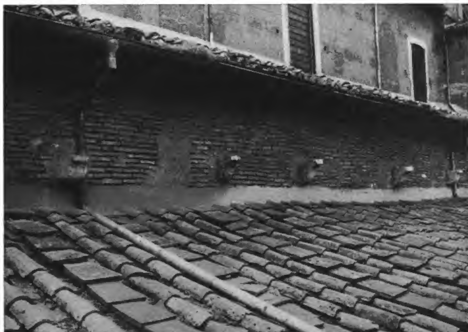
Fig. 126. SS. Nereo ed Achilleo, Wall of north aisle
